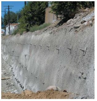
into place using a separate grout line, whereas hollow bars may be drilled and grouted simultaneously by using a sacrificial drill bit and by pumping grout down the hollow bar as drilling progresses.
